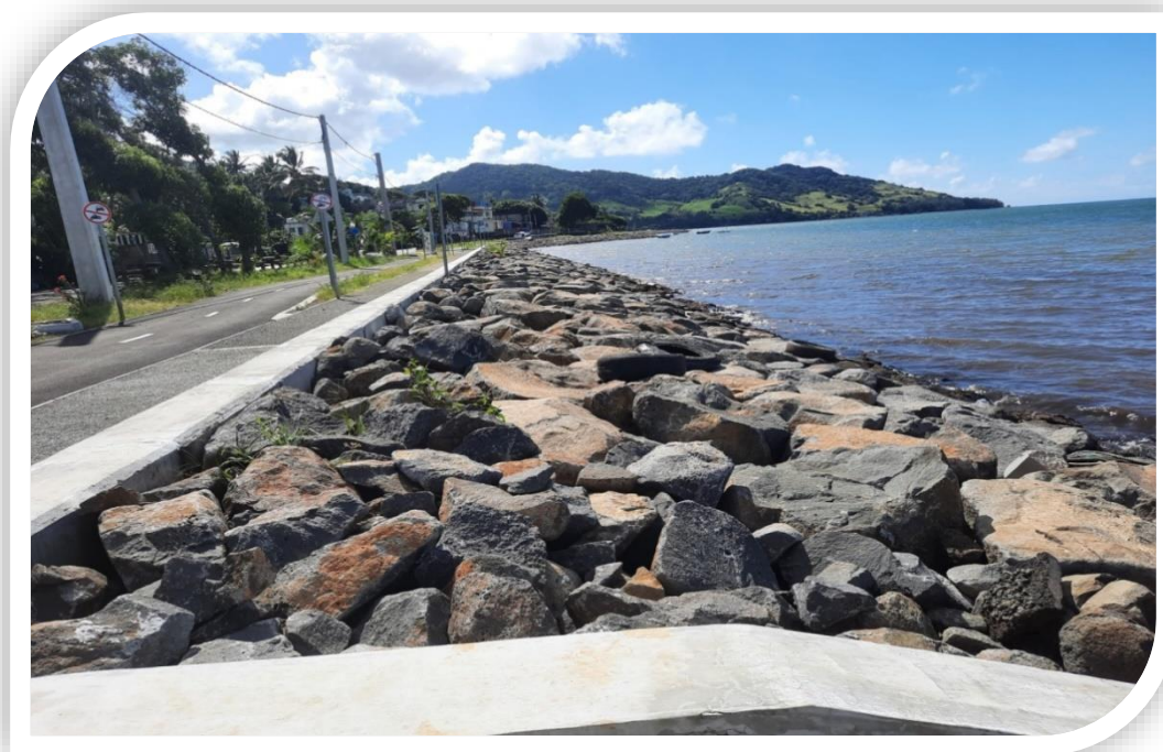
Rock revetment at Providence - Bois des Amourettes
